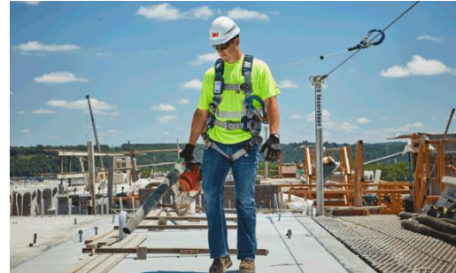
Figure 58 – Fixed static line
