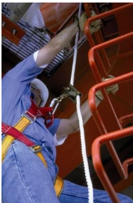
Figure 11 – Temporary rope line with rope grab
