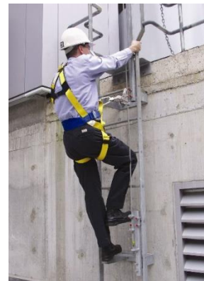
Figure 12 – Permanent wire line with wire grab
