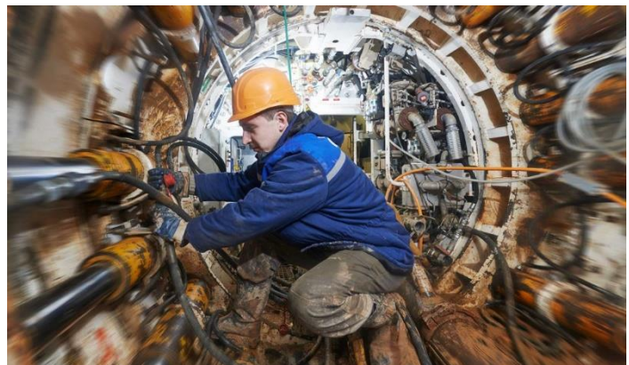
Figure 20 – Working in a Confined Space
