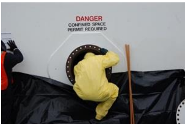
Figure 19 – Entering a Confined Space
