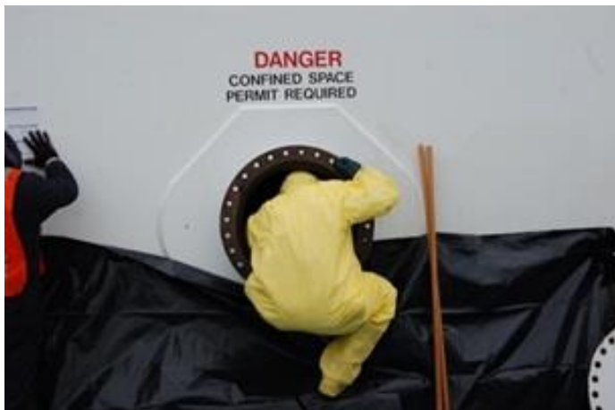
Figure 24 – Entering a Confined Space
