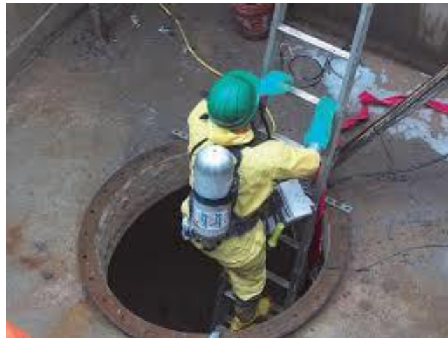
Figure 26 – Exiting from a Confined Space
