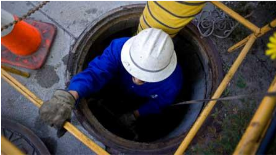
Figure 23 – Entering a Confined Space
