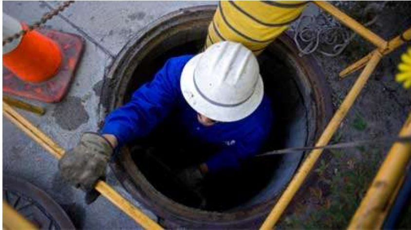
Figure 23 – Entering a Confined Space
