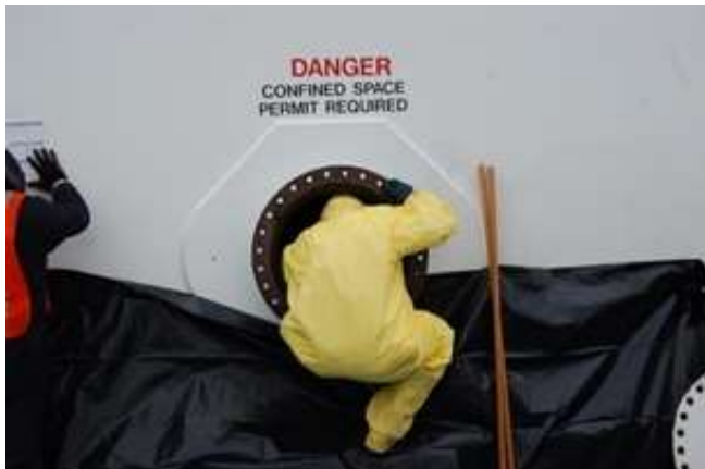
Figure 24 – Entering a Confined Space
