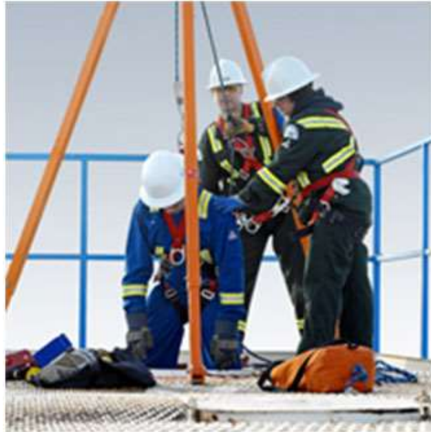
Figure 8 – Entry using a tripod
