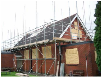
Tube and Coupler Scaffolds
